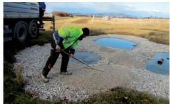
Fig: Building of a pond. The pond is sealed with pond liner.
