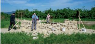
Fig.: Fundament and professional construction of a dry stone wall.
